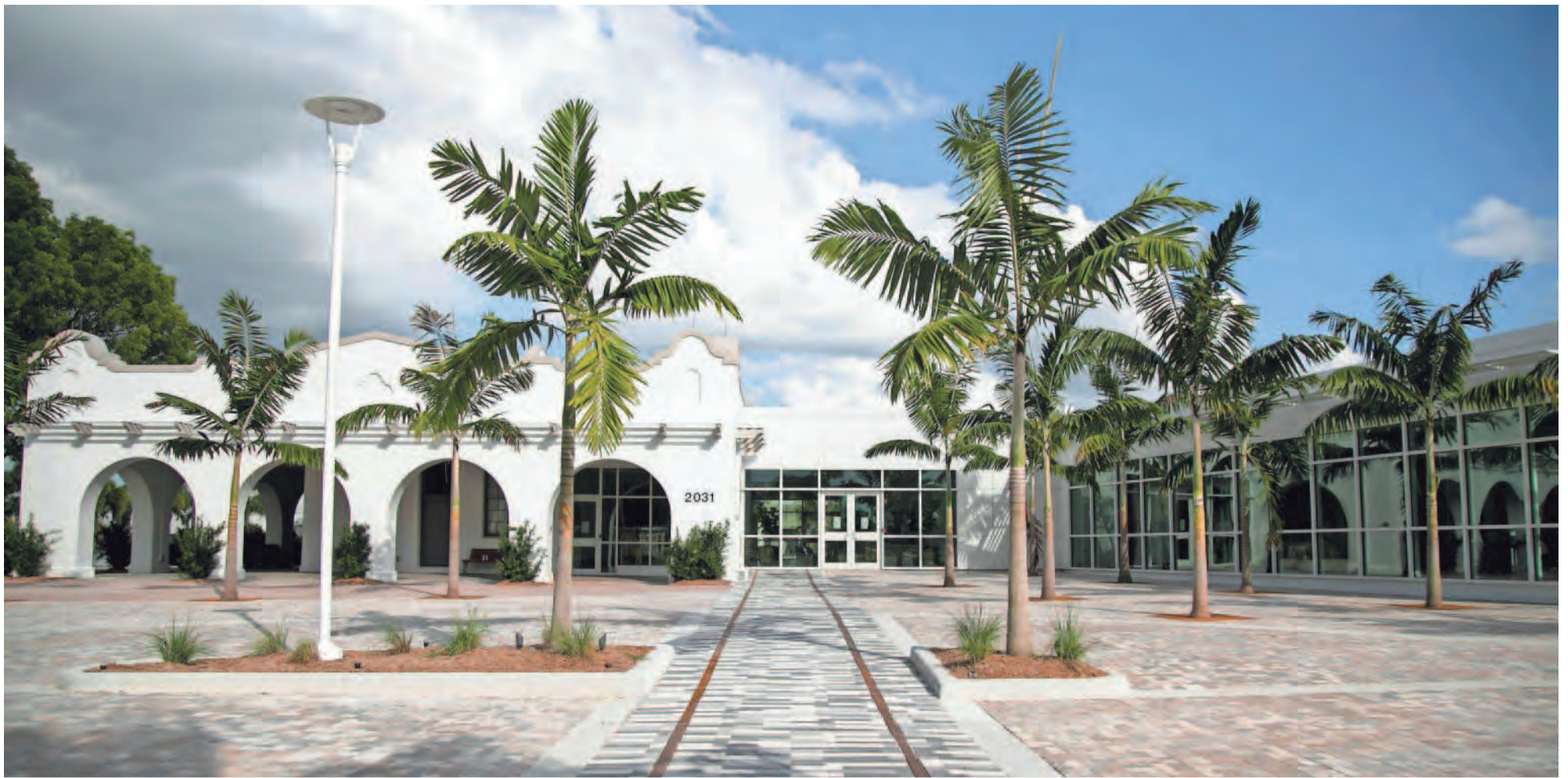
The Collaboratory in downtown Fort Myers is a public-private partnership with the Southwest Florida Community Foundation and the City of Fort Myers. The building includes the historic train depot and a new LEED addition that includes the Foundation's regional headquarters and a shared space for the community and tenants. AMANDA INSCORE/THE NEWS-PRESS
